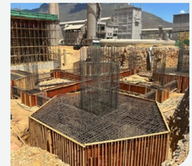
PCC preheater tower.
