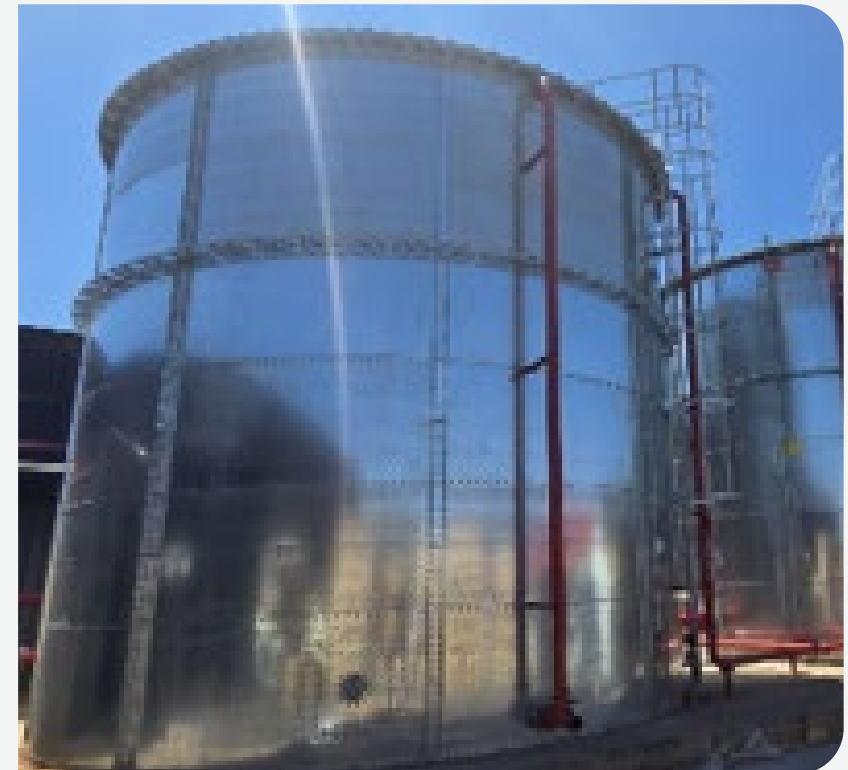
Installation of water-efficient systems for manufacturing clients.
